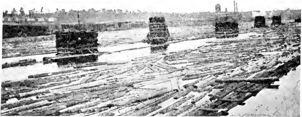
FIG. 142. — Piers placed in a River to hold Storage Booms. Minnesota.
